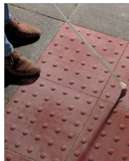
TACTILE PAVING - TYPE 1 TYPE 1 - RED TACTILE PAVING AT ALL SIGNALISED PEDESTRIAN CONTROLLED CROSSINGS ONLY. SCALE = 1:20
