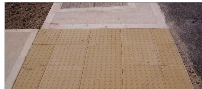
TACTILE PAVING - TYPE 2 TYPE 2 - BUFF TACTILE PAVING AT ALL DISHD CROSSINGS. SCALE = 1:20
